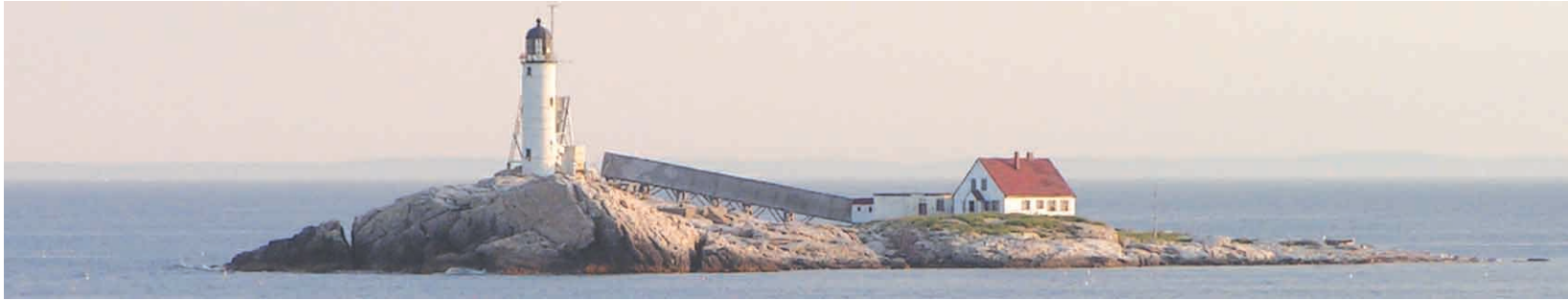
TO BE REPAIRED — Like many lighthouses, White Island requires repairs to remain standing against the elements.
