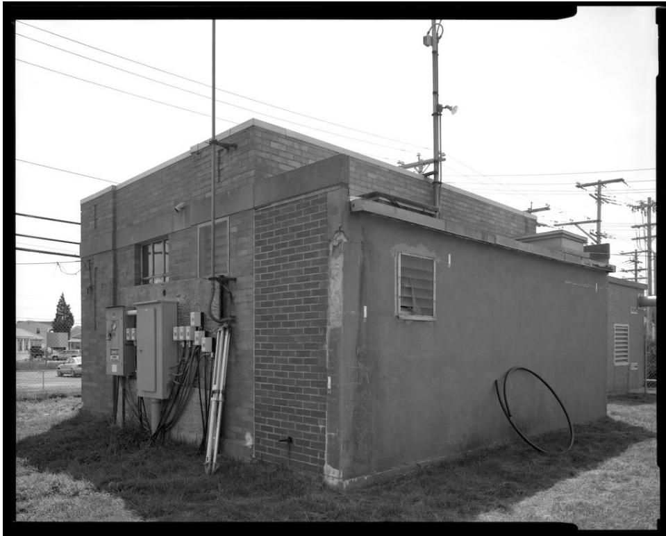
NH-718-2: East elevation and rear addition (1968). Looking southwest.
